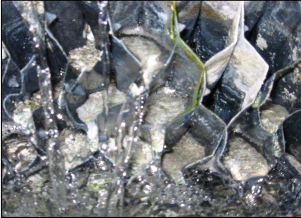
Scale accumulation near water level on media.
