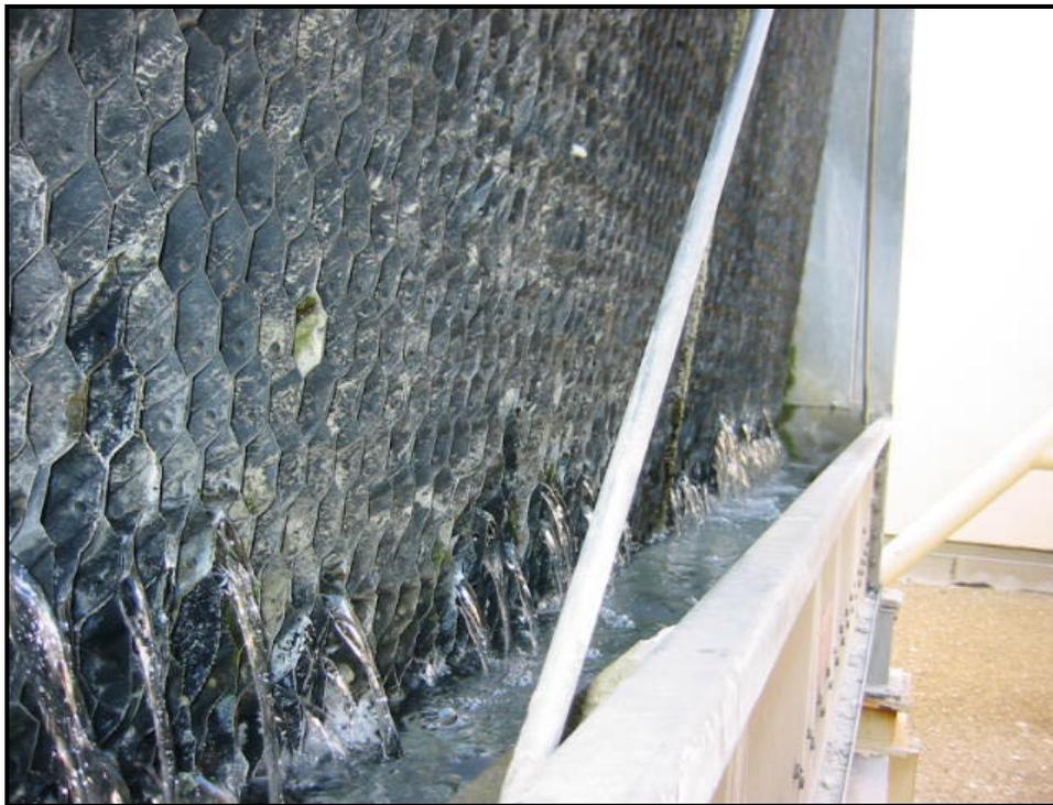
**Scale accumulation causing water spouts prior to treatment
