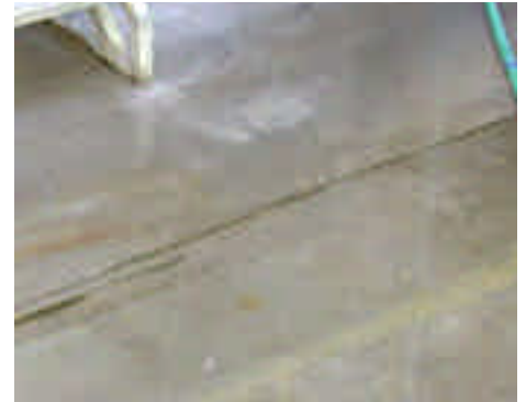
After 60 days of treatment, the area floors were clean and slight remaining scale was soft and powdery.
