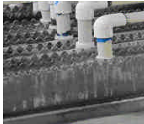
30 days after treatment, scale was partially removed and dissolved away with normal use.
